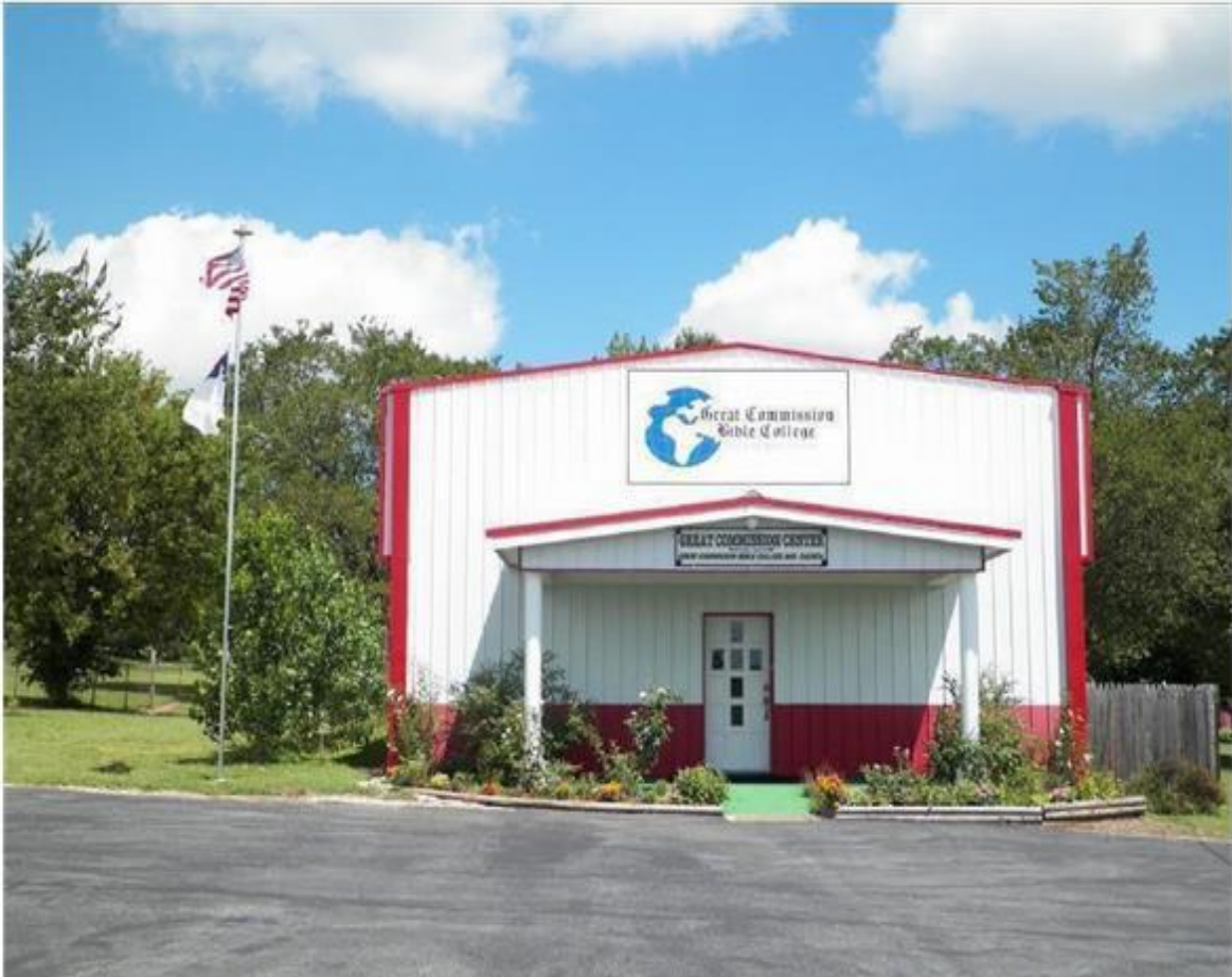
Photo above is GCBC Administration Building
